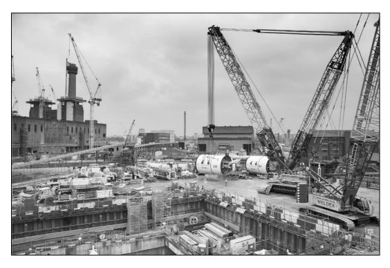
A major milestone in the construction of the Northern Line Extension was reached this week with the lowering of two giant tunnel boring machines 20 metres below ground in Battersea, ahead of tunnelling starting in March.
